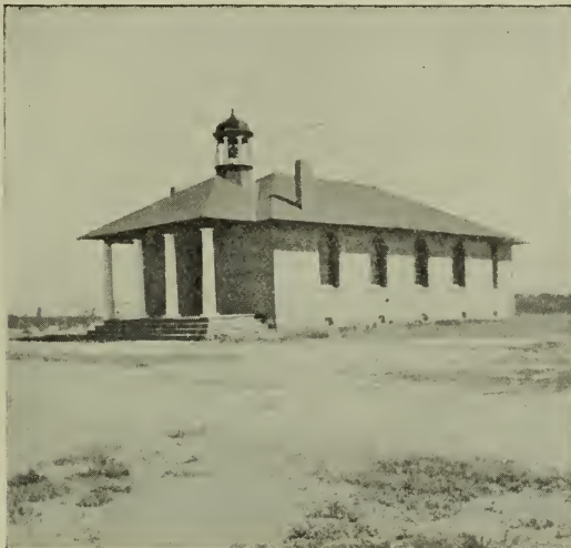
JOHN ELIOT MEMORIAL CHAPEL, TUCSON, ARIZ.
